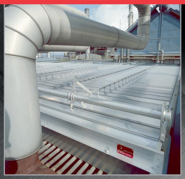
Louvers can be operated either manually or automatically, using pneumatic or electrical actuator-positioners.
